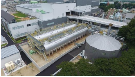
Kyoto City Southern Clean Center
